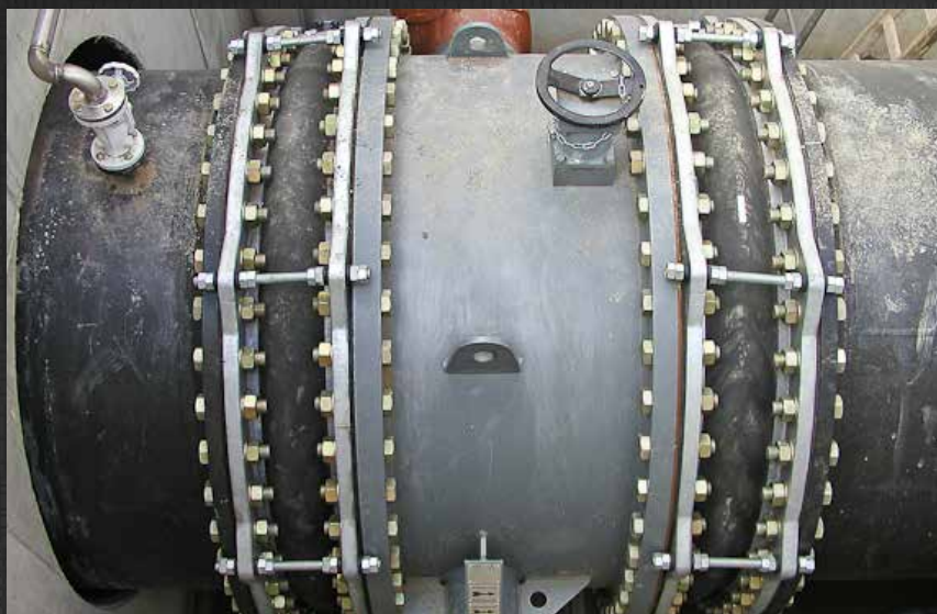
Rubber expansion joints type U110M as dismantling joints NB 2000, 6 bar
