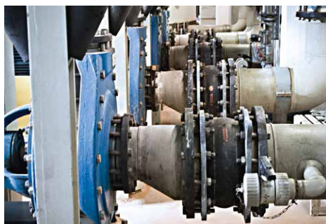
Expansion joints with swivel flanges, type D110A pumping header installation NB 300, operating pressure 10 bar ▶ page 121
