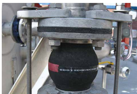
Lateral expansion joint, type U110R on the pump pressure side in a paper mill NB 50, 10 bar ▶ page 187
