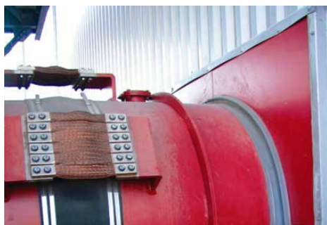
Pipe penetration seal and clamped EPDM rubber expansion joint penetration seal made from silicone rubber with open seam for afterwards closing on site ▶ page 127
