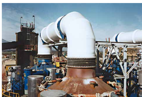
Universal expansion joint, type U152A with PTFE lining in a GRP pipe in a copper mill NB 2000, -0.17 bar, earthquake movements all sides \pm 150 mm ► page 79
