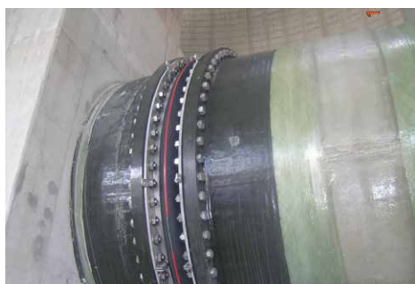
Universal expansion joint U110A in a cooling tower NB 3100, 4 bar, axial / lateral \pm 40 mm ► page 75
