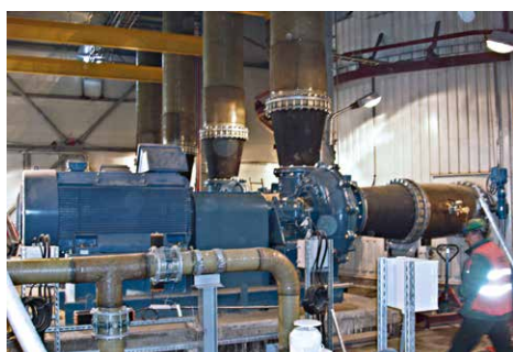
Conical expansion joints, type U300A on the suction and discharge side of a gypsum slurry pump in a desulphurization unit of a power plant ► page 87
