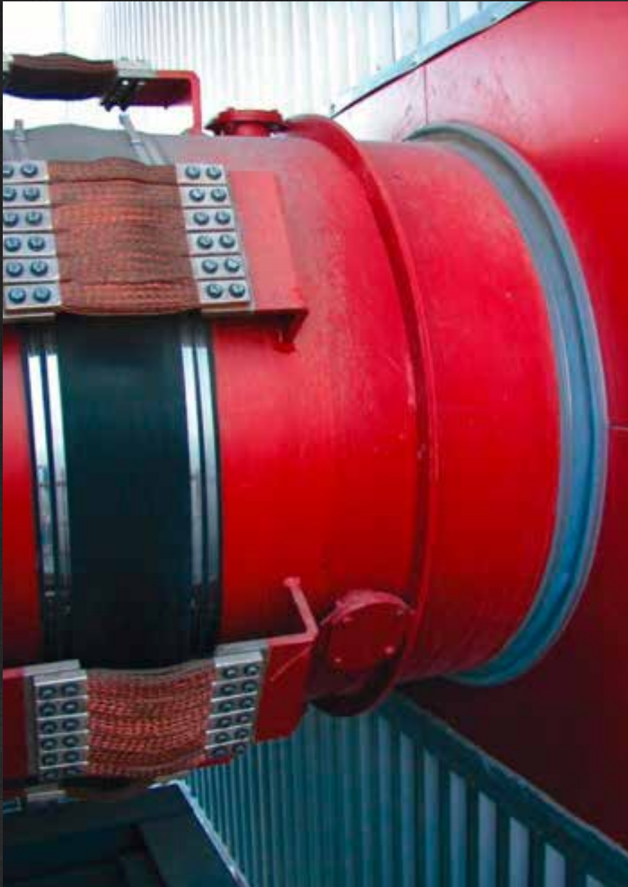
Pipe penetration seal and clamped EPDM rubber expansion joint penetration seal made from silicone rubber with open seam for afterwards closing on site
