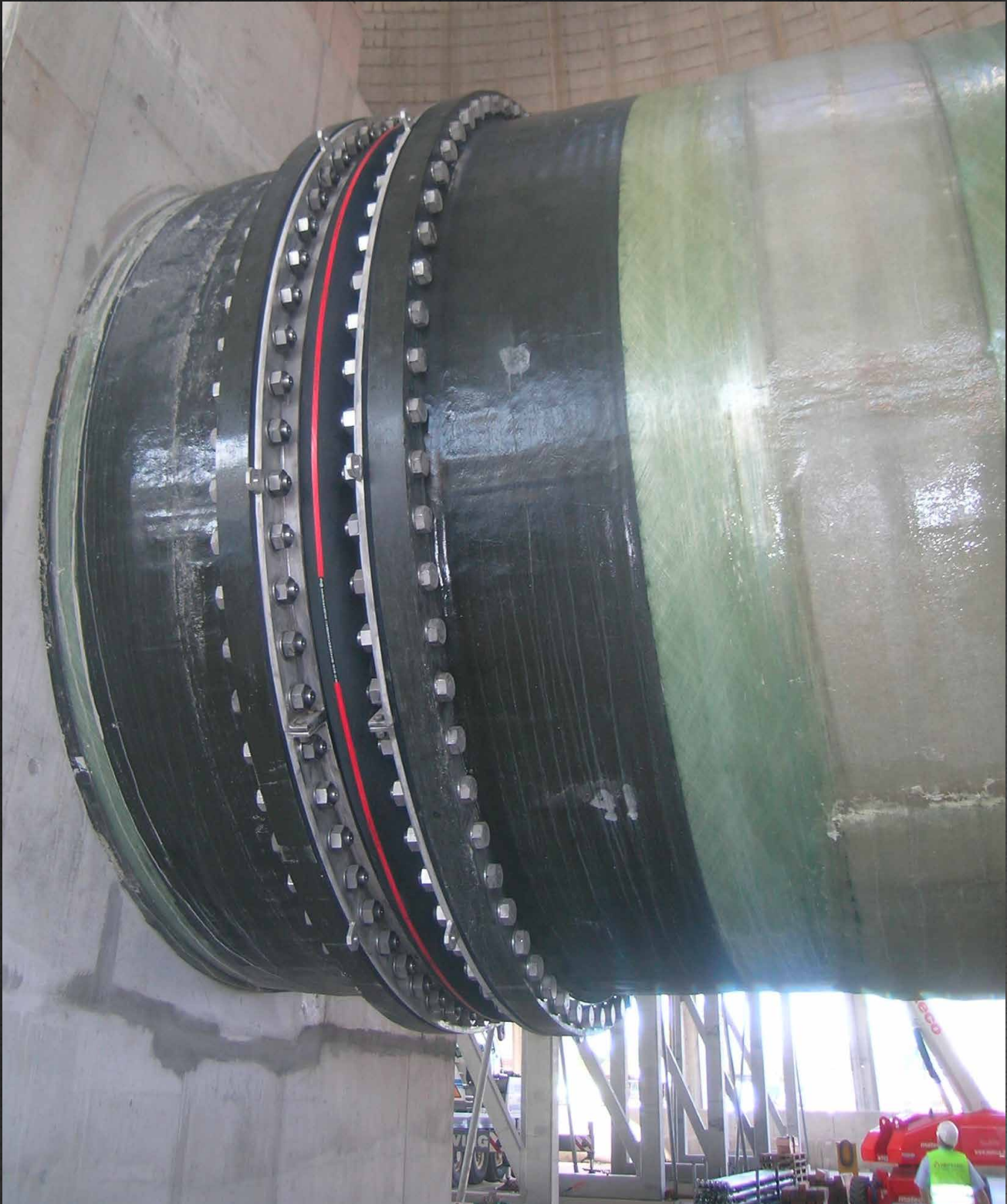
Universal expansion joint U110A in a cooling tower NB 3100, 4 bar, axial / lateral \pm 40 mm
