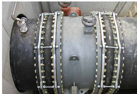
Lateral expansion joints used as dismantling joints in a valve pit NB 2000, PN6 ▶ page 17
