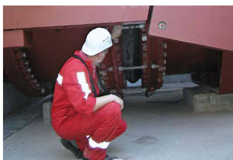
Lateral expansion joint, type U110M in the cooling water system of a coal-fired power plant NB 2600, 4 bar ► page 83
