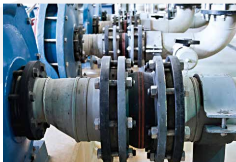
Universal expansion joint, type D110A on the suction side of quenching water pumps in a waste incineration plant NB 150, 16 bar ▶ page 105
