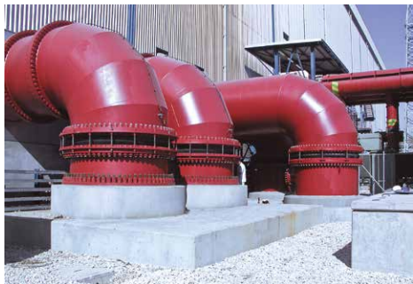
Lateral expansion joint type U110M in the cooling water system of a coal-fired power plant. NB 2600, 4 bar ▶ page 17
