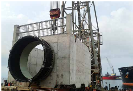
Type U110A universal expansion joint Cooling water intake basin NB 3600 ▶ page 45
