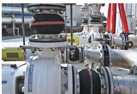
Universal and lateral expansion joint on a lye pump suction and discharge side NB 125, 5 bar ▶ page 189
