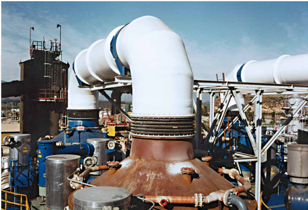
Universal expansion joint, type U152A with PTFE lining in a GRP pipe in a copper mill NB 2000, -0.17 bar, earthquake movements all sides \pm 150 mm
