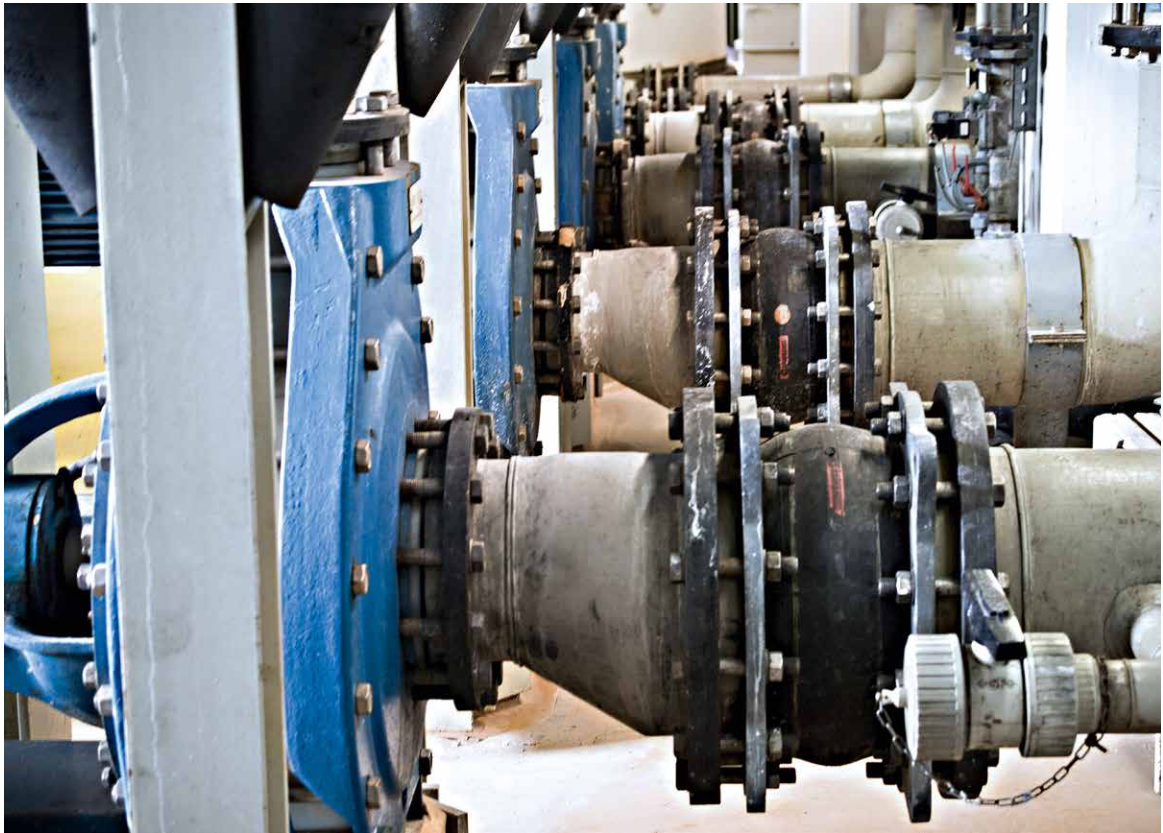
Expansion joints with swivel flanges, type D110A pumping header installation NB 300, operating pressure 10 bar
