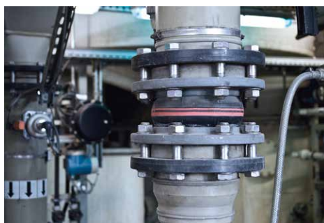
Universal expansion joint, type D110A in a plastic pipe of a paper plant NB 150, design pressure 6 bar ▶ page 120
